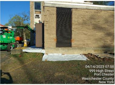
Photograph 3 -Abatment of asbestos- and PCBcontaining caulking at the former power plant using hand tools, view facing northeast.
