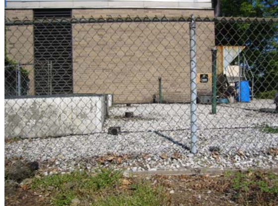
Photo #2: UST Installation
