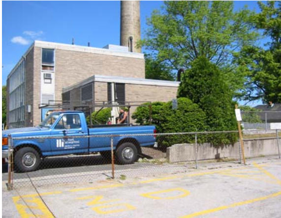
Photo #1: Boiler Room / Generator Room
