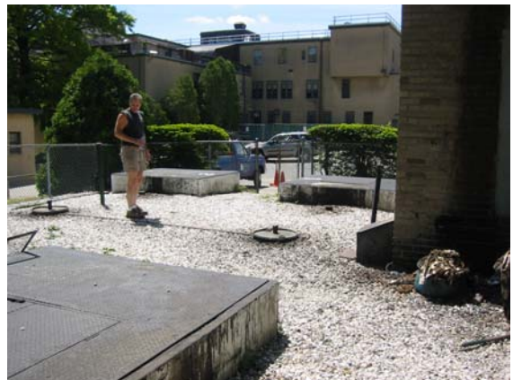
Photo #3: UST Installation
