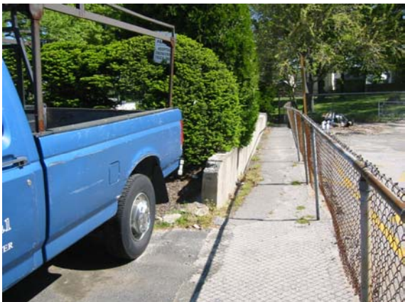
Photo #6: Side of UST installation
