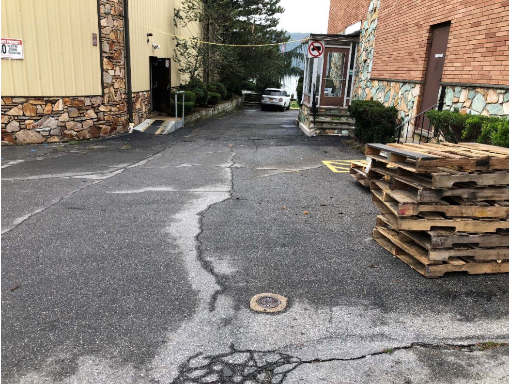
Photograph No. 5: Photograph of the on-site groundwater monitoring well associated with the 5,000-gallon No. 2 fuel oil UST grave (facing west).
