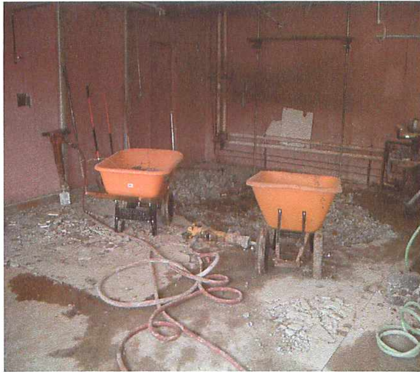
Photo 1, View of the initial excavation area
