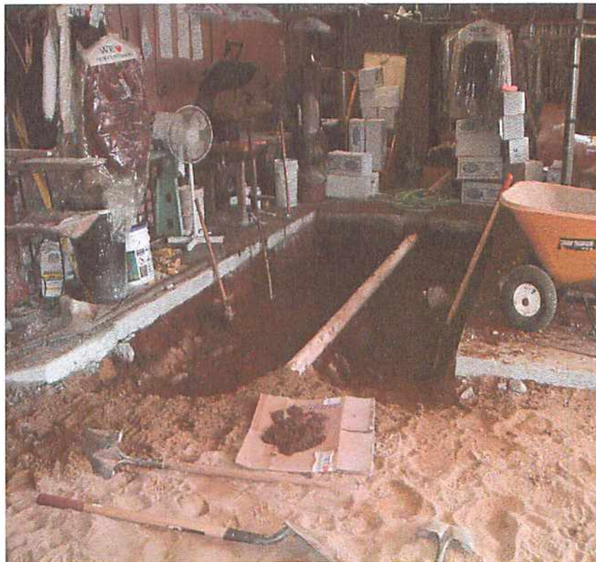
Photo 3, View of the additional excavation area
