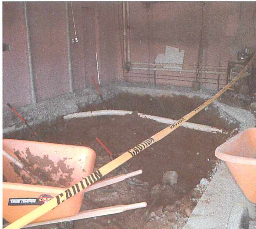
Photo 2, View of the initial excavation area
