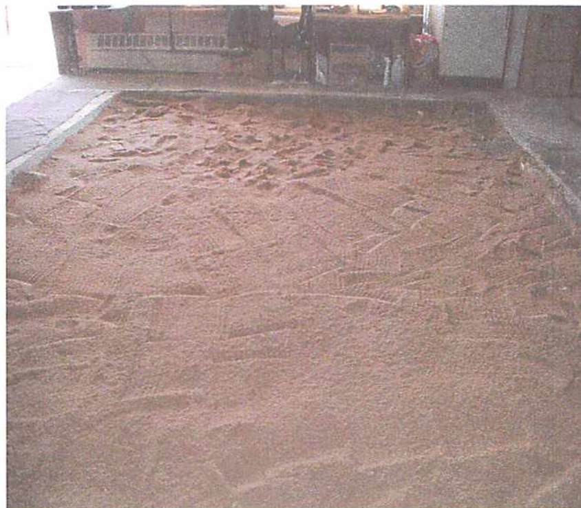
Photo 4, View of the completed excavation area
