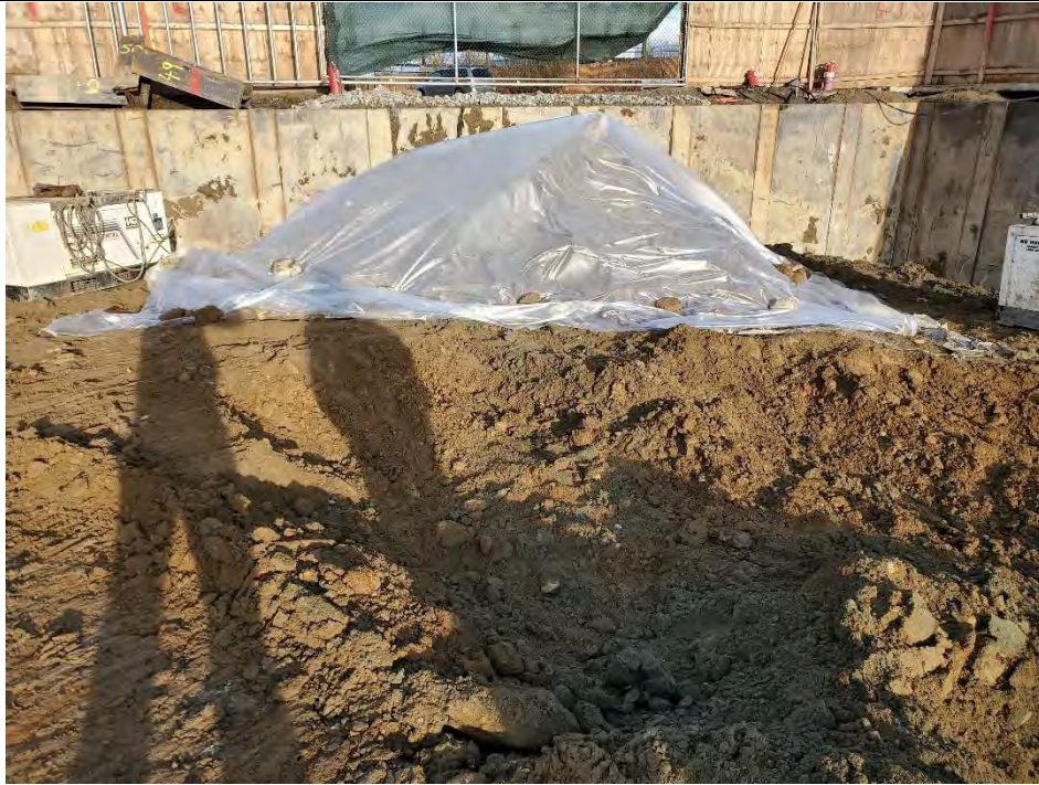
Photo 3: View of UST in Excavation and Stockpiled Soil.
