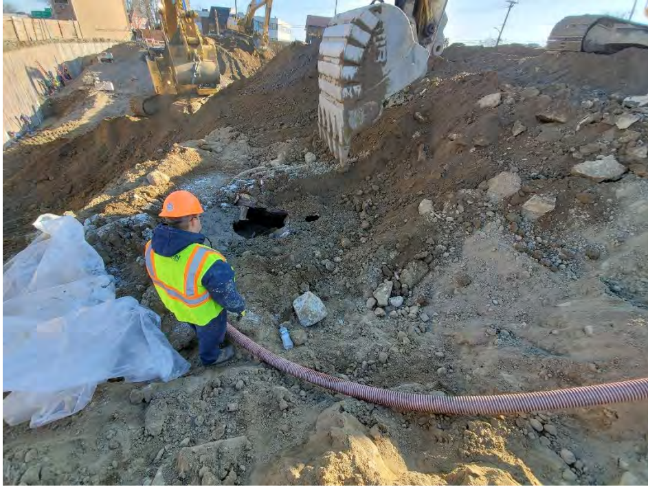
Photo 5: View of UST-3 Exposed
