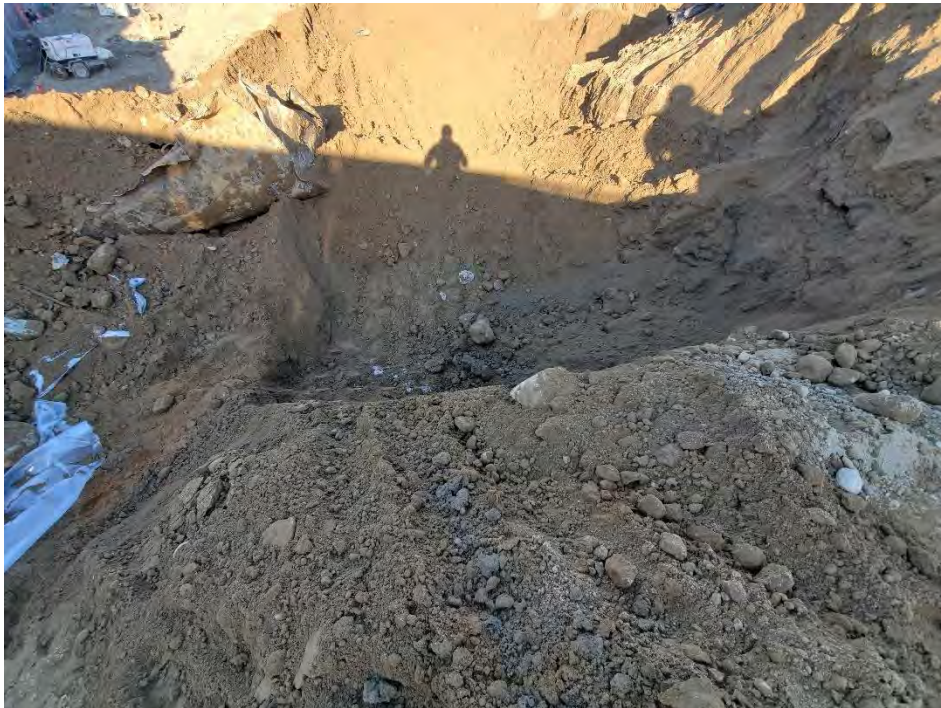
Photo 8: View of UST-3 Excavation
