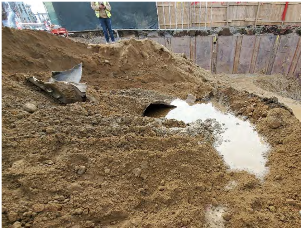
Photo 4: View of UST-3 in Place (Minor Water Spillage).
