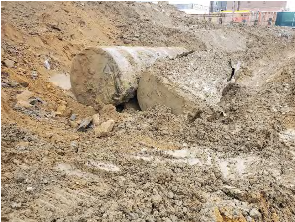
Photo 2: View of UST-1 and UST-2 Removed. Top Open Exposing Concrete
