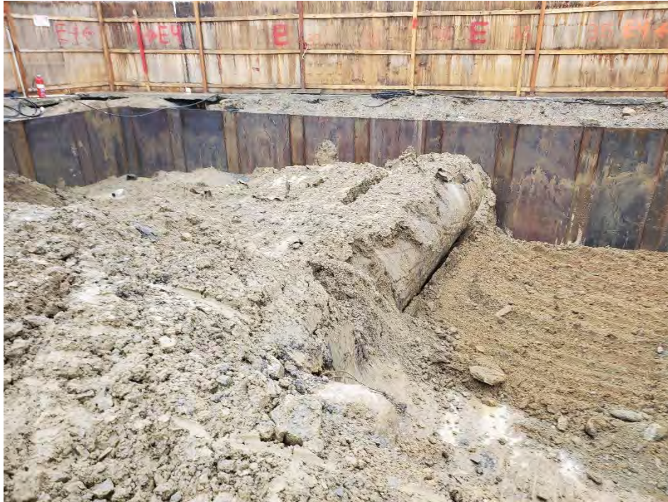
Photo 1: View of UST-1 and UST-2 in Place
