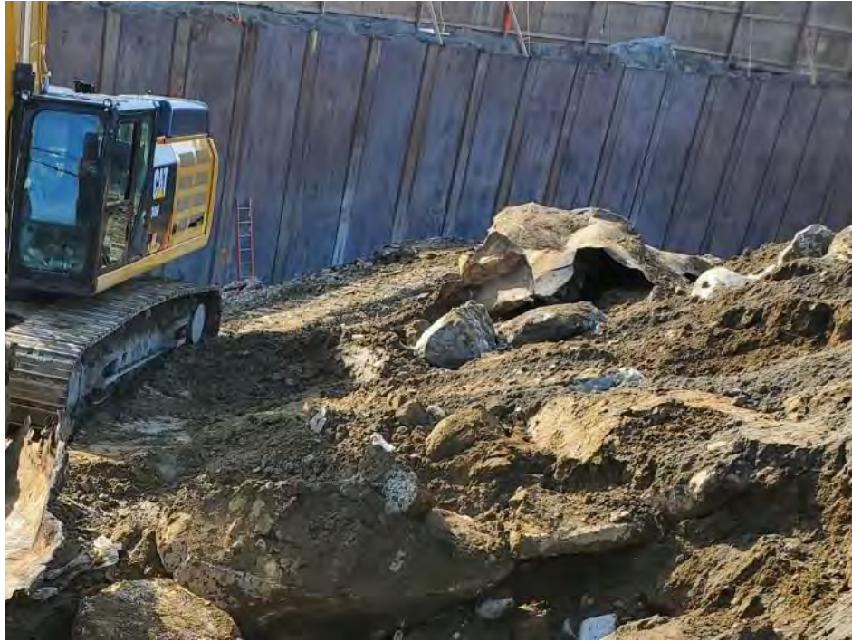
Photo 7: View of UST-3 Removed
