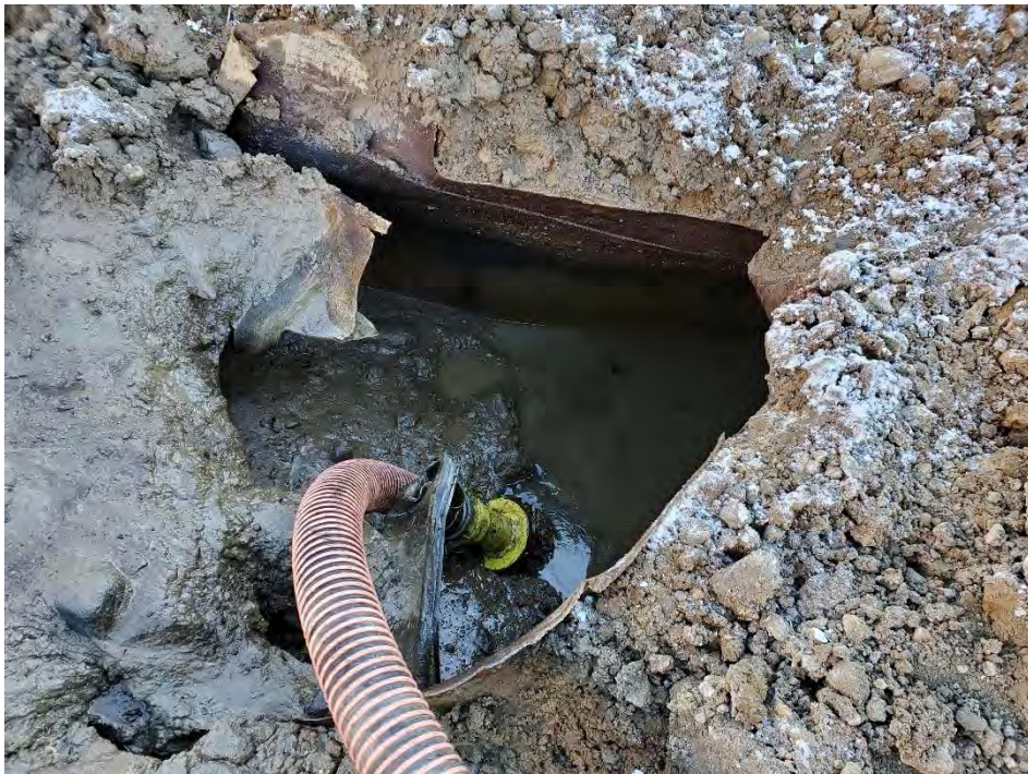
Photo 6: View of UST-3 Vacuum Truck Pumping Water Content
