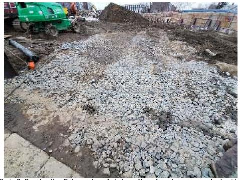
Photo 2: Construction Entrance heavily laden with sediment, recommend refreshing
