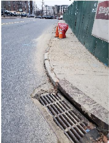
Photo 4: Sediment deposited on southwest corner of Garden Street and Cottage Place from water line discharge earlier in the week. Recommend replacing catch basin controls due to punctured fabric.
