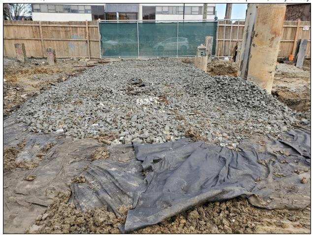
Photo 10: Construction Entrance (Taken after inspection was completed)
