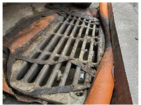
Photo 2: View of inlet protection practice installed over catch basin on northwest end of Cottage Place.
