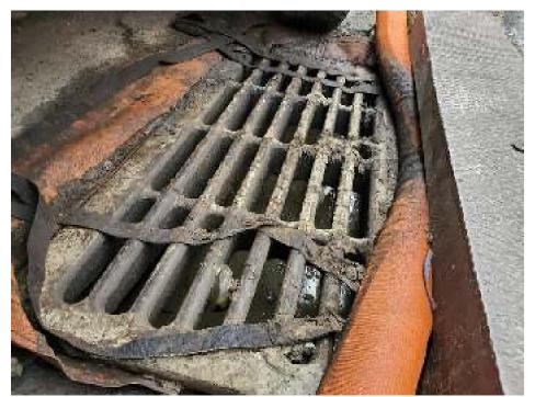
Photo 2: View of inlet protection practice installed over catch basin on northwest end of Cottage Place. Replacement of the inlet protection is recommended due to oily condition and accumulated sediment to properly filter all drained sediment in inlet protection practices.
