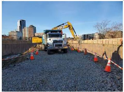
Photo 1: Tracking pad/construction entrance to Cottage Place. Recently placed stone is sufficiently cleaning tracked soils from vehicle tires. No modifications recommended.
