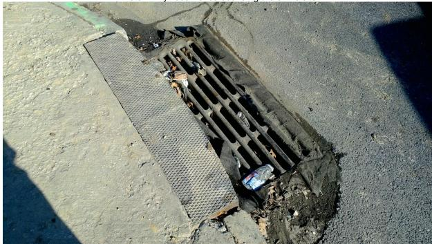
Photo 2: Filter Fabric added to corner curb inlet
