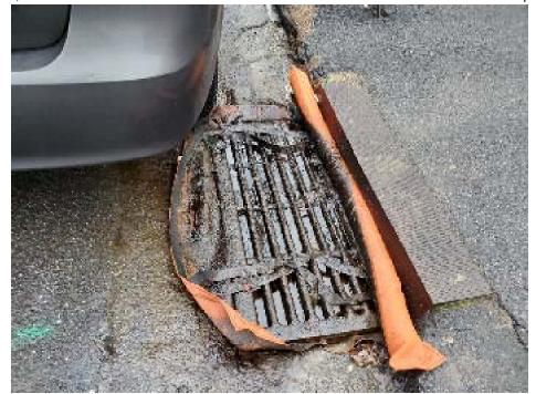
Photo 3: View of inlet protection practice installed over catch basin on northwest end of Cottage Place.
