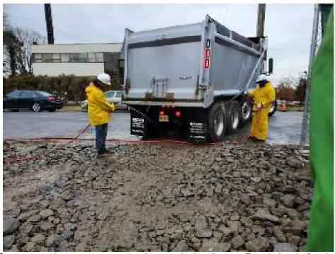
Photo 2: Contractor using water sprayer to clean tracked sediment off truck tires before leaving Site.
