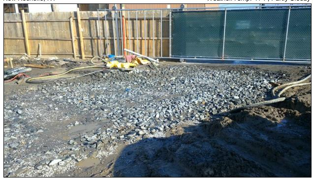
Photo 3: Construction Entrance/Tracking Pad; This entrance will be decommissioned and a new location for the entrance and tracking pad will be utilized.
