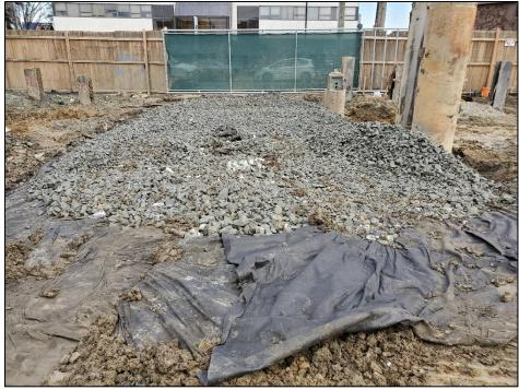
Photo 4: Relocated Construction Entrance/Tracking Pad; Currently in progress and was not utilized during the time of inspection.
