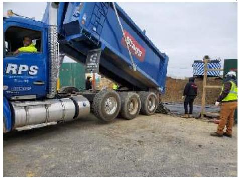
Photo 1: Construction of tracking pad on southern border of site, adjacent to existing parking lot
