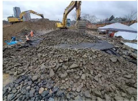
Photo 1: Construction entrance on Cottage Place. Contractor installing stone over filter fabric per SWPPP
