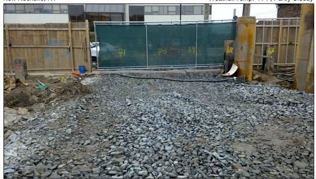
Photo 3: Relocated Construction Entrance.
