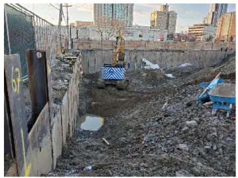
Photo 4: Sheets and piles acting as sediment barrier along vast majority of the perimeter of the Site.
