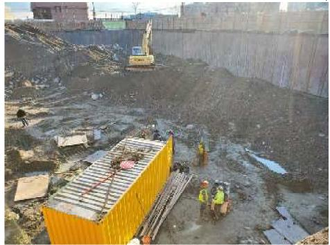
Photo 3: Sheets and piles acting as sediment barrier along vast majority of the perimeter of the Site.
