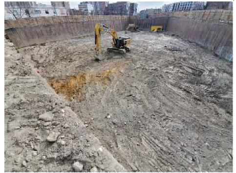
Photo 1: Excavation area currently inactive, view from Cottage Place. Photograph taken on 3/18/20. Sheets and piles acting as sediment barrier along vast majority of the Site perimeter.
