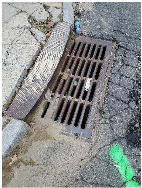
Photo 5: Catch basin on northwest corner of Garden Street and Cottage place. Recommend installing inlet protection controls.
