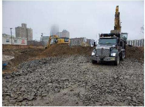
Photo 3: View of active soil stockpiles and truck-loading operations on northwest end of Site, facing south.
