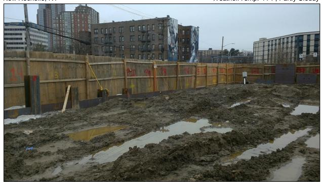
Photo 1: Construction Plywood Fence and Sheet Piles along Garden Street.
