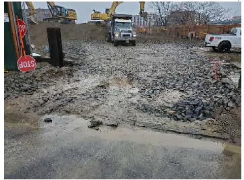
Photo 1: Western-most construction entrance on Cottage Place. Recommend placing filter fabric and refreshing stone on the tracking pad to prevent soil pumping and off-Site tracking.
