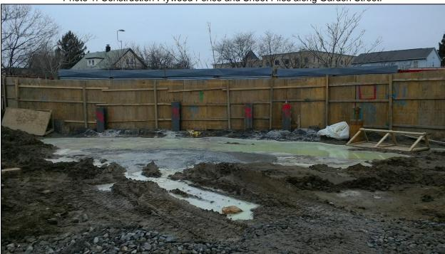
Photo 2: Observed Concrete Washout Area; There should be a designated and properly constructed concrete washout area.
