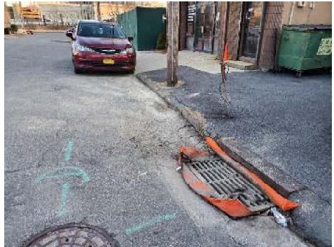
Photo 3: View of inlet protection practice installed over catch basin on northwest side of Cottage Place. Further modification of installation and removal of accumulated sediment is recommended to properly filter all drained sediment in inlet protection practices
