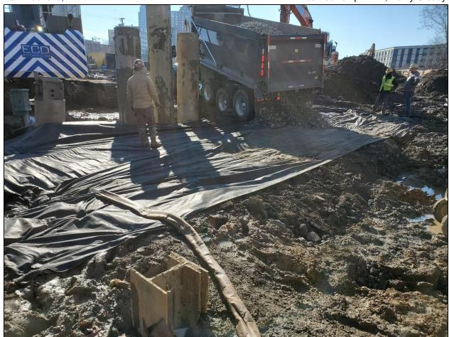
Photo 9: Construction Entrance Relocation in progress (Taken after inspection was completed)
