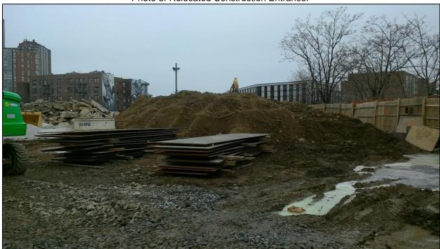
Photo 4: Observed Stockpile on-site; If left inactive for 14 days, a silt fence is recommended to be placed around its edges to prevent sediment erosion.
