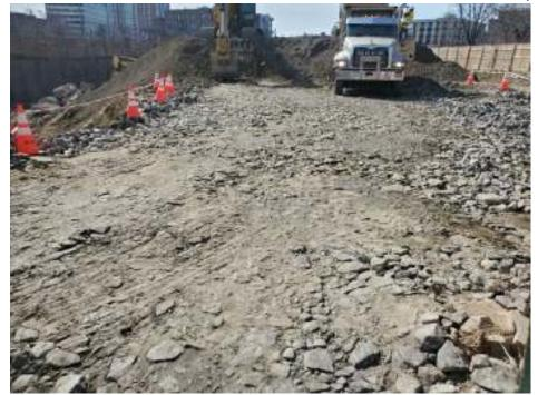
Photo 1: Tracking pad/construction entrance to Cottage Place. Deposited sediment is insufficiently cleaning tracked soils from vehicle tires. Recommend refreshing stone at entrance.
