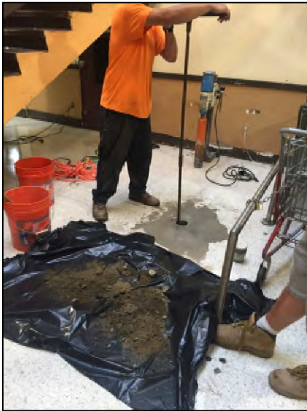
Photograph 1: Advancing SB-7 using hand auger.
