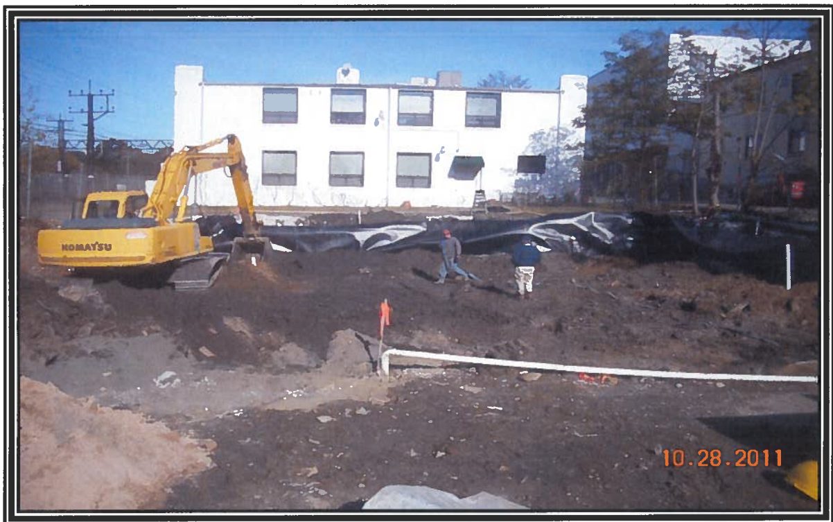
Photograph taken during backfilling and polyethylene barrier installation
