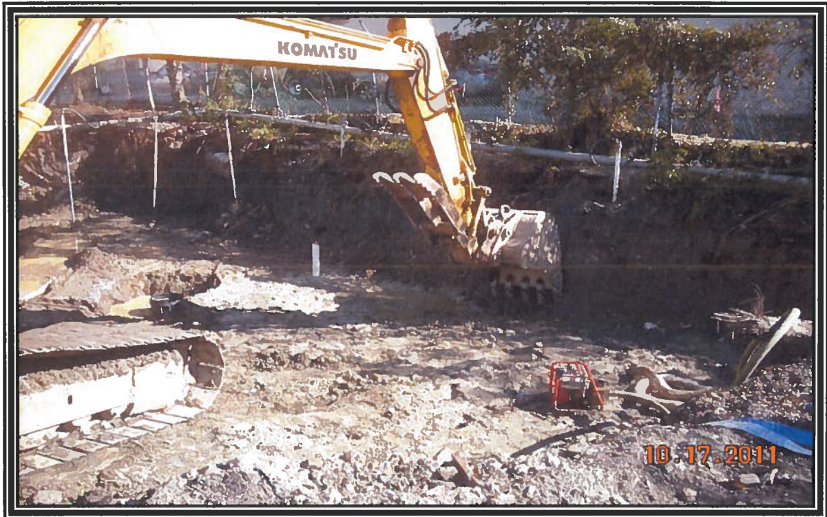
Photograph taken during soil excavation activities
