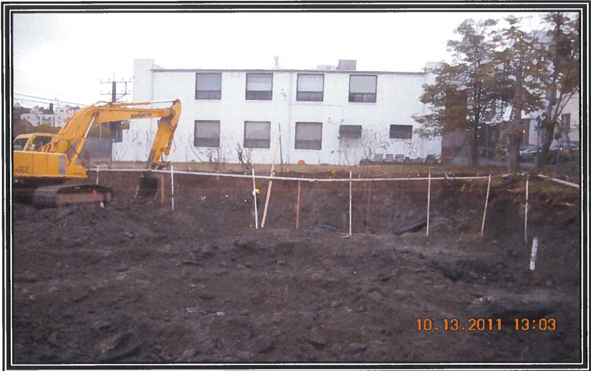
Photograph taken during dewatering and soil excavation activities
