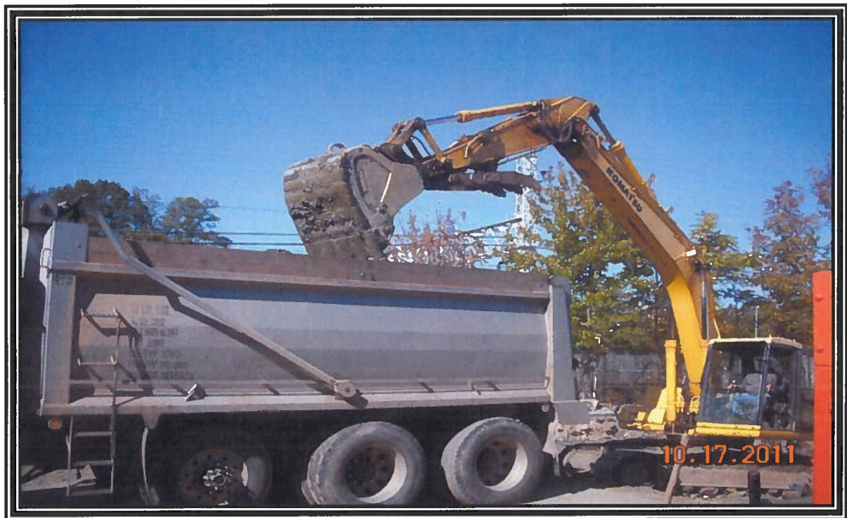
Photograph taken during soil loading and removal activities
