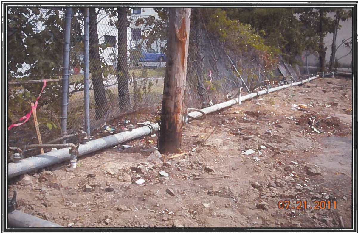
Photograph taken of dewatering wells and header pipe
