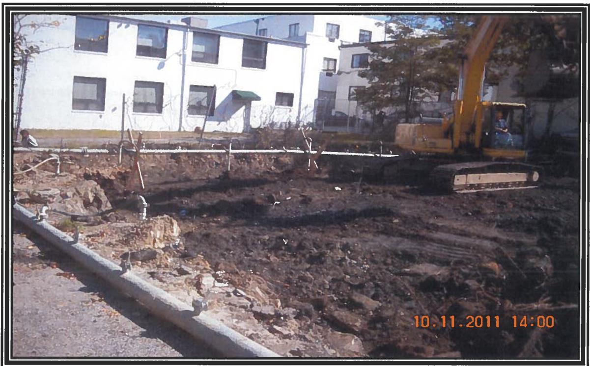
Photograph taken of dewatering wells and header pipe during excavation activities
