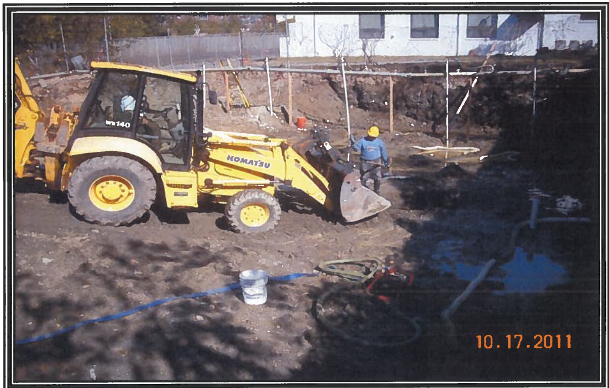
Photograph taken during soil excavation activities
