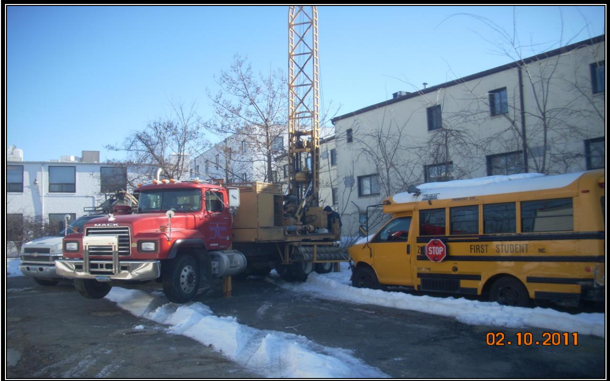
Photograph taken during the installation of monitor wells MW-1 through MW-4
