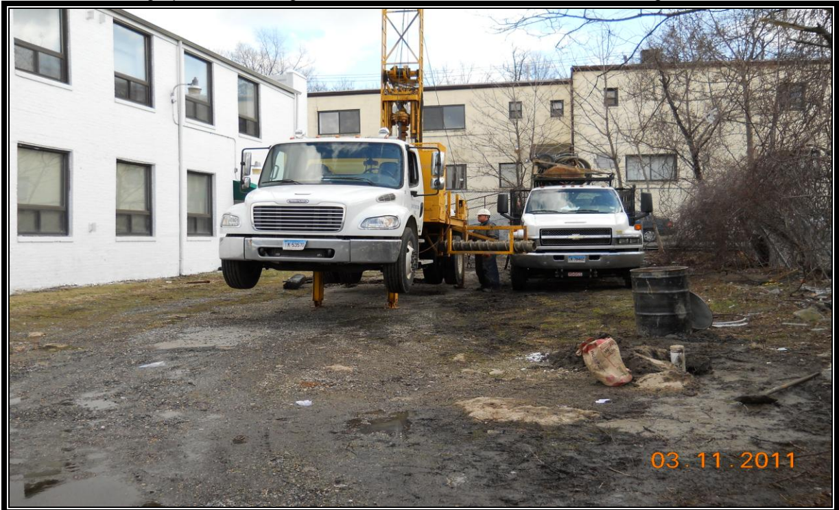
Photograph taken during installation of monitor wells MW-5 through MW-7
