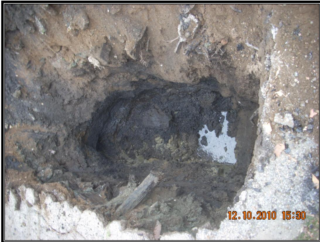
Photograph of impacted groundwater at TP-1
