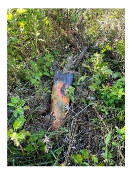
Photo 3 Damaged Site groundwater monitoring well MW-1 from unknown event – to be decommissioned.
