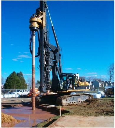
AUGER MIXING WITH TRACK MOUNTED DRILL RIG
