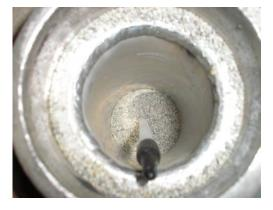
Hydrating bentonite to assure proper seal
