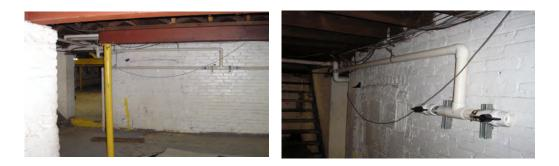
Basement piping manifold for each for North and South basement trenching
