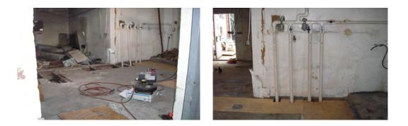
Installation of manifold for all SVE wells and SSDS
