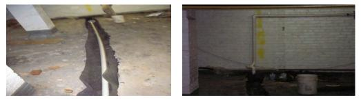
Trenching for SSDS in Basement of Schmukler's Cleaners
