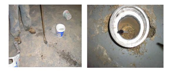
Hand installation of permanent vapor point
