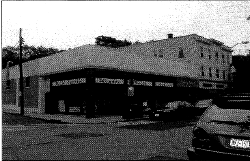
SUBJECT PROPERTY, VIEW TO THE SOUTHEAST.
