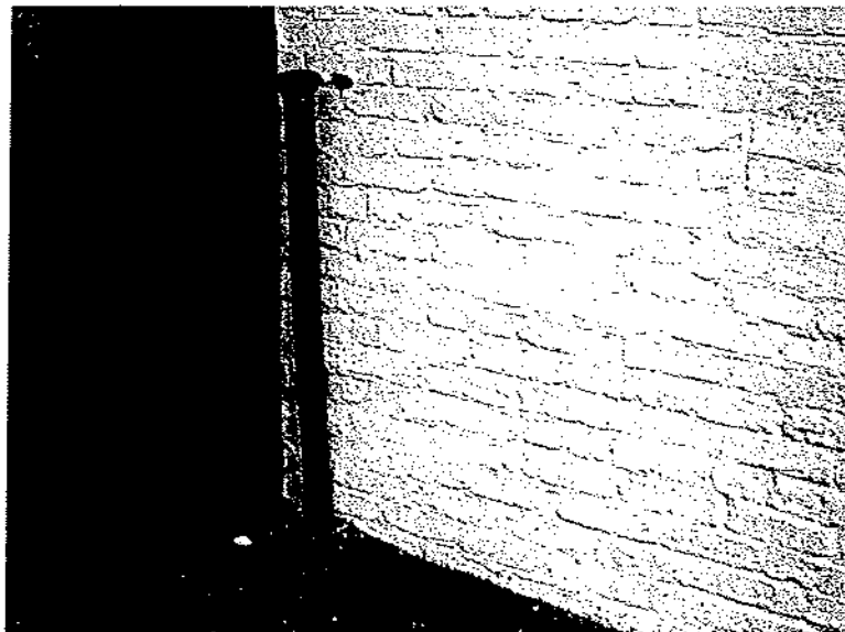
Close-up of Fuel Oil Underground Storage Tank Vent Line
