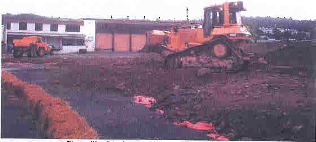
Photo #9 - Placing clean soil cover - northern area.
