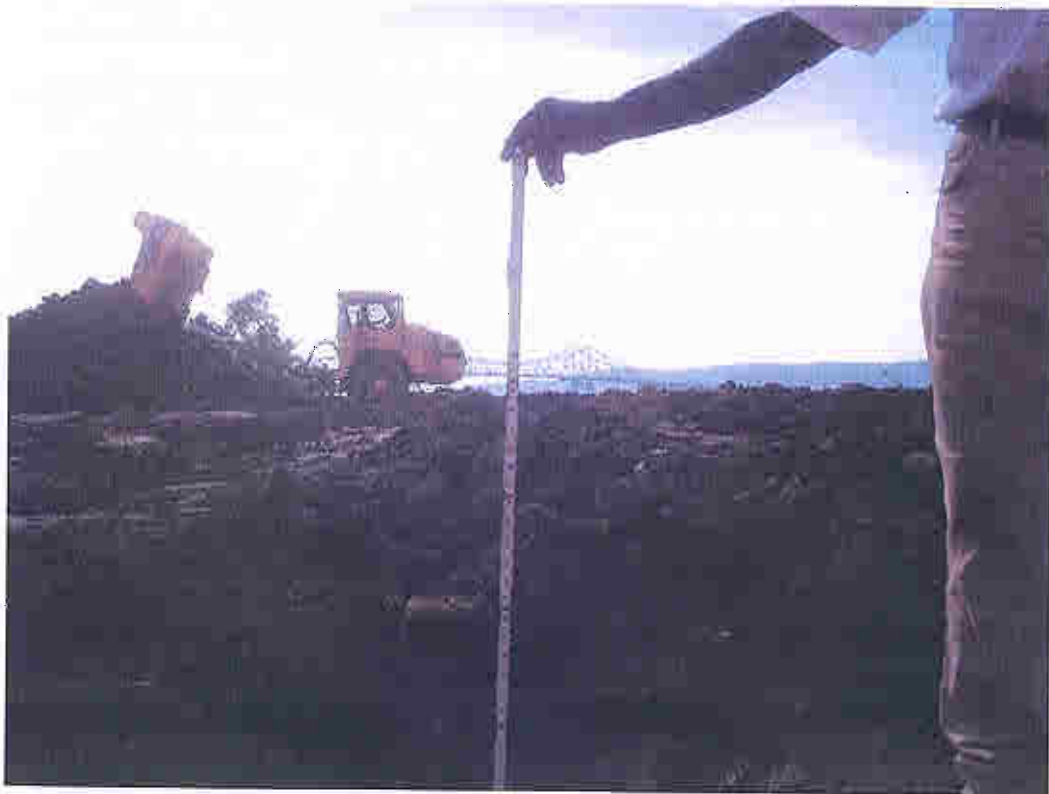
Photo #10 - Verifying minimum thickness of clean soil cover.
