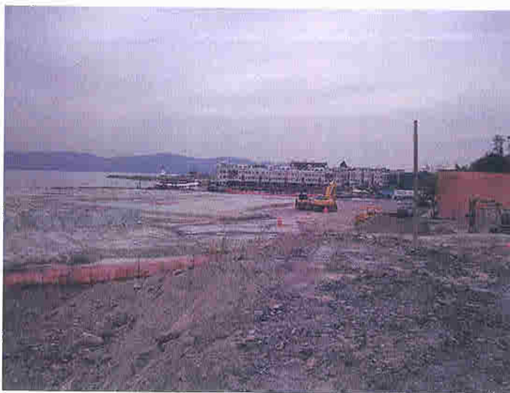
Photo #12 - Clean soil cover looking north.
