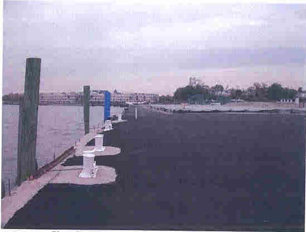
Photo #1 - Asphalt pavement at river front looking north.
