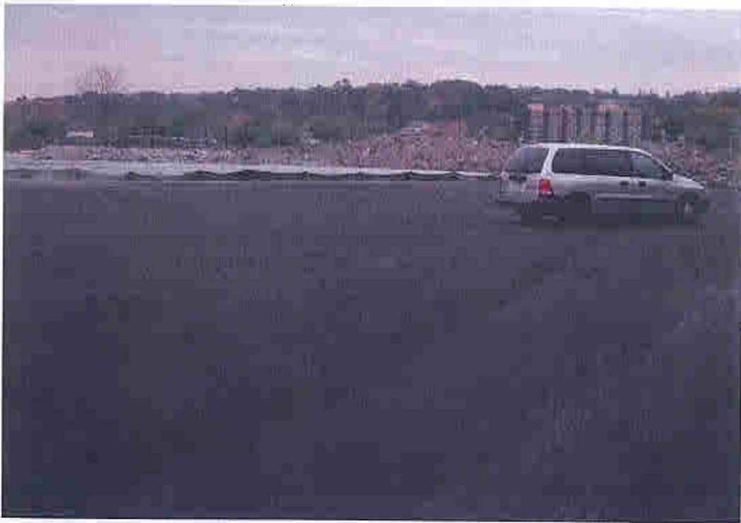
Photo #3 - Asphalt pavement in southwest area looking east.
