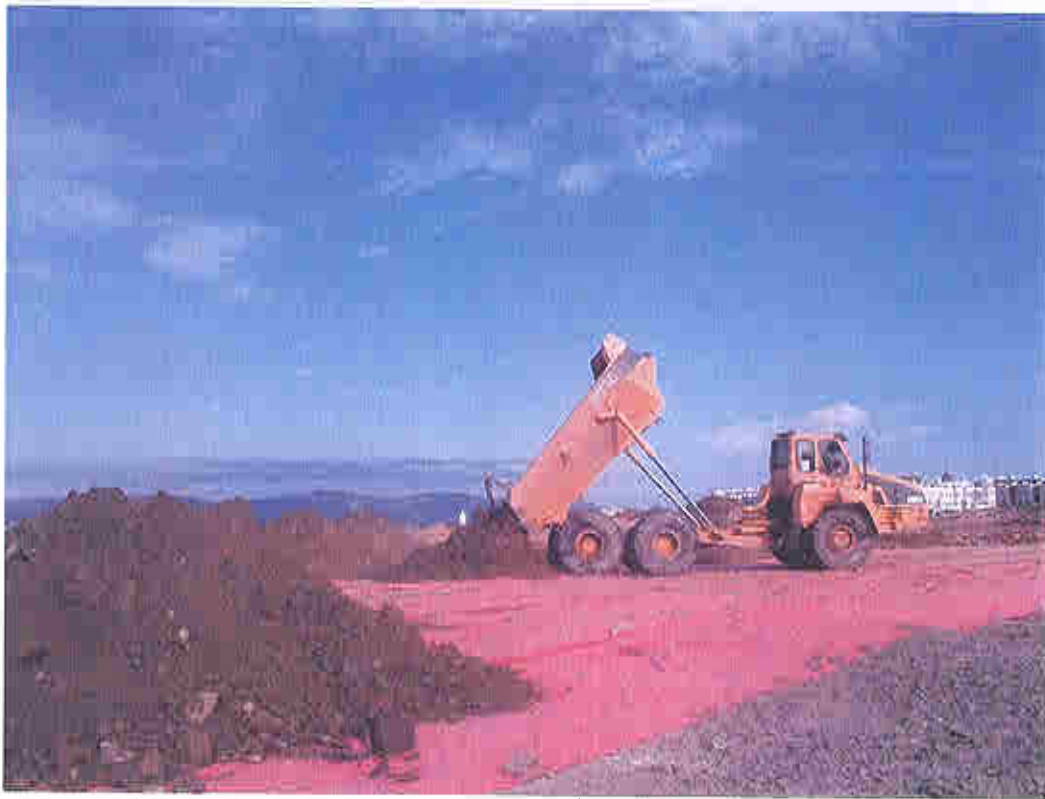
Photo #4 - Dumping clean soil onto demarcation layer.
