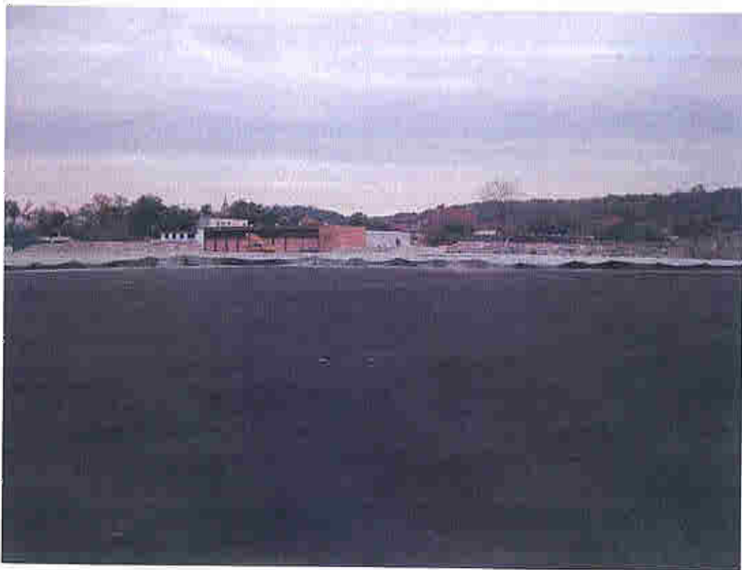
Photo #2 - Asphalt pavement in southwest area looking northeast.
