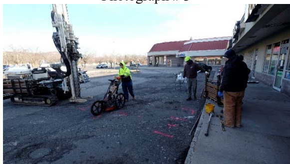
GPR Survey at MW-4
