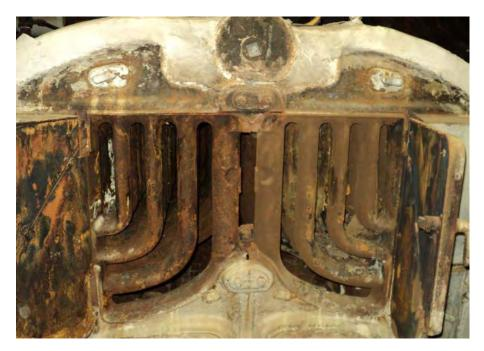
6. Boiler with asbestos thermal wrap.
