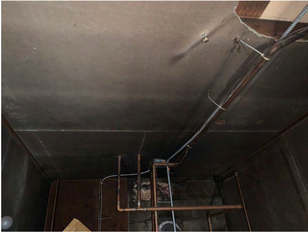
(ACM Cement Panels on Walls & Ceiling in Room 1)
