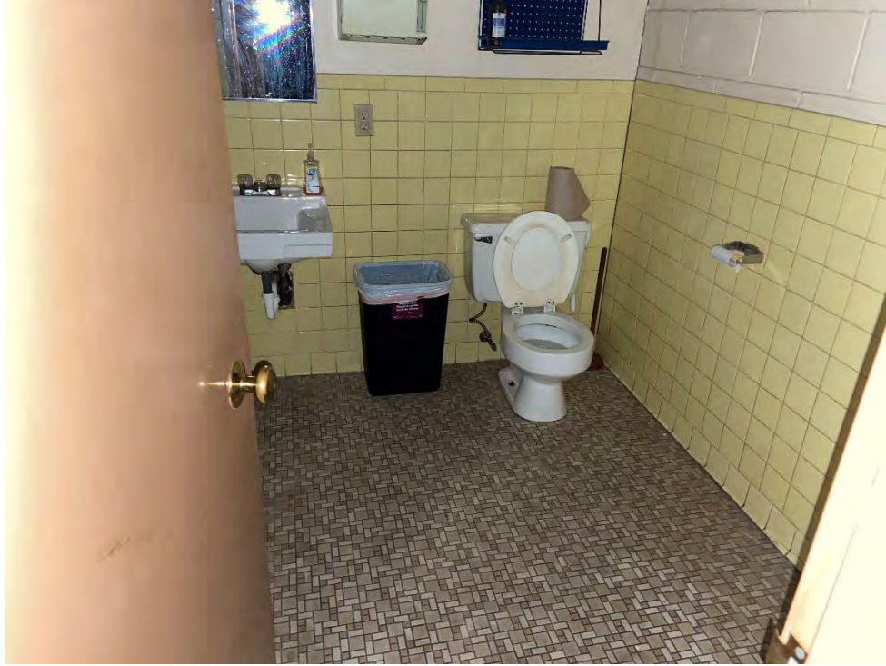
(ACM Ceramic Tile Adhesive Behind Ceramic Tiles in Bathroom 4)
