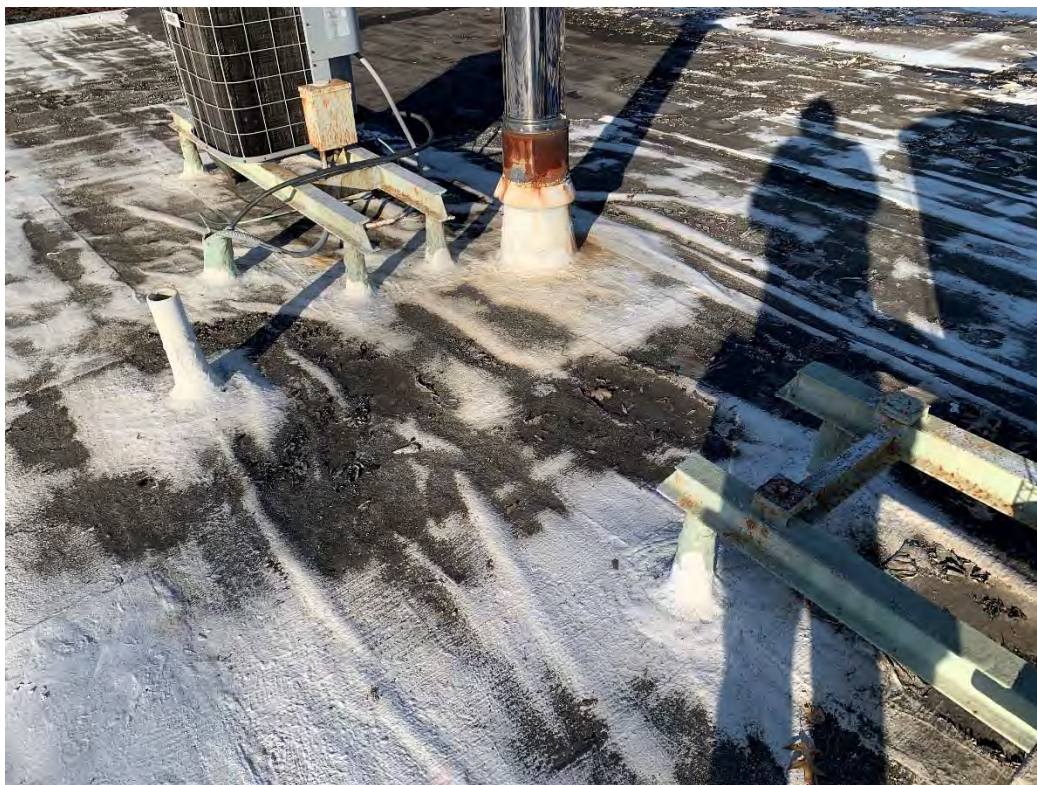
(ACM Flashing Tar and ACM Pitch Pocket Tar on Roof)
