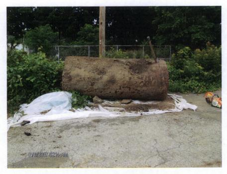
1000-gallon fuel oil UST facing south from the southern side of building. One of the two tanks removed from Site 2.
