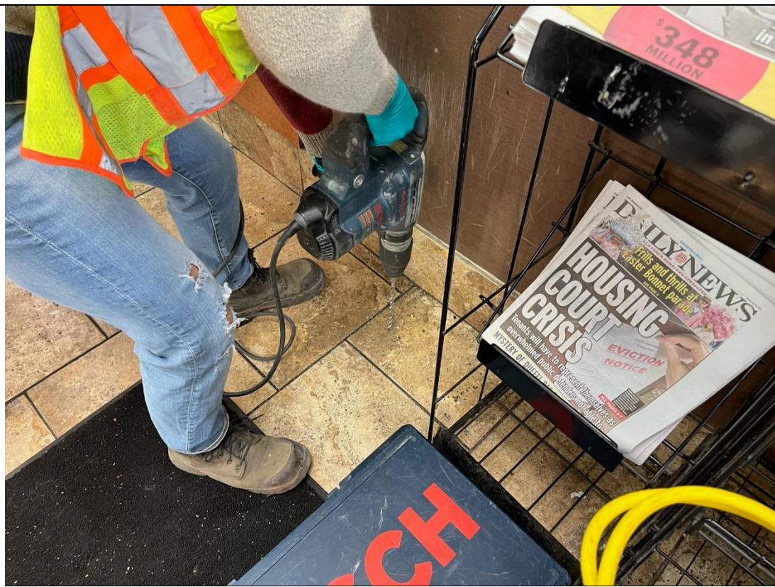
Photo 1 – View of Langan installing a temporary sub-slab soil vapor sampling point within the bagel shop tenant space, facing north.
