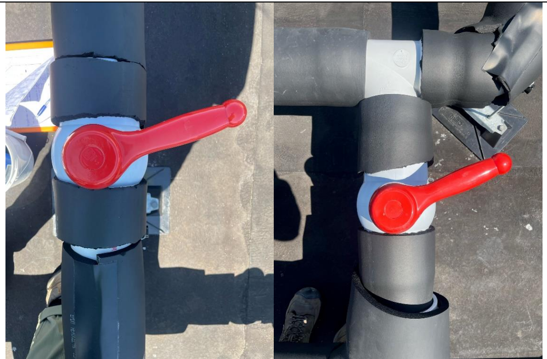
Photo 4 – View of grocery sub-header valves at approximately 75% closed upon departing the site, facing northwest (left) and facing northeast (right).
