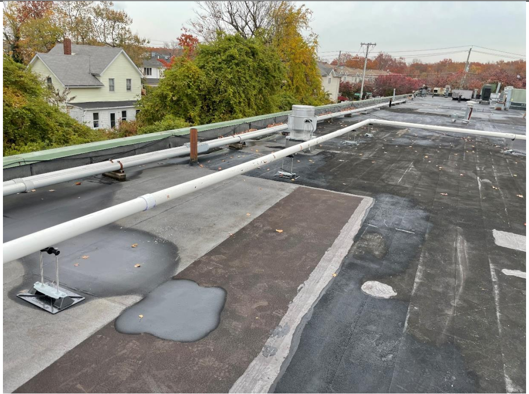
Photo 3 – View of newly installed subheader line (associated with VEP-18, VEP-19, VEP-21, VEP-22, VEP-25 and VEP-26) running towards the main header, facing north.
