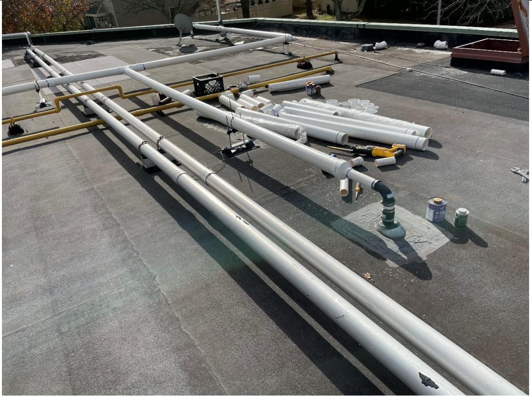
Photo 3 – View of VEP-11 connected to the 4-inch PVC subheader line, facing south.
