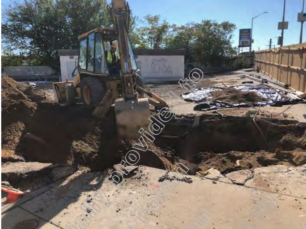
Excavating remaining three unknown tanks
