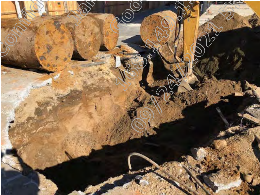
Unknown tank excavation
