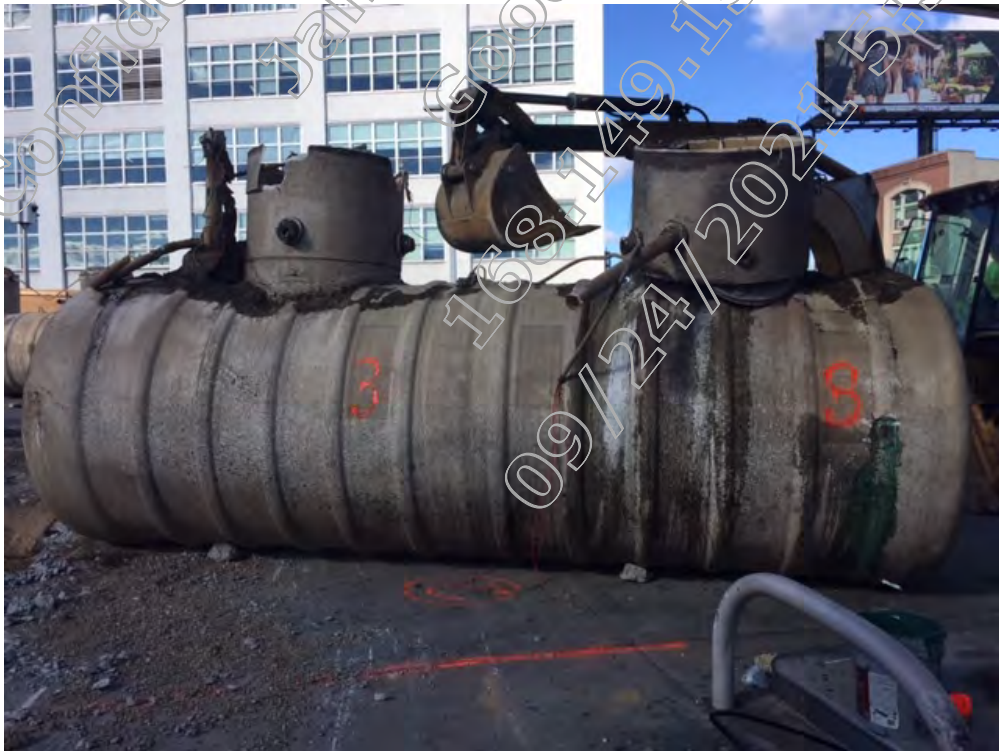
Condition of tank #3 (4,000-gallon double walled fiberglass)
