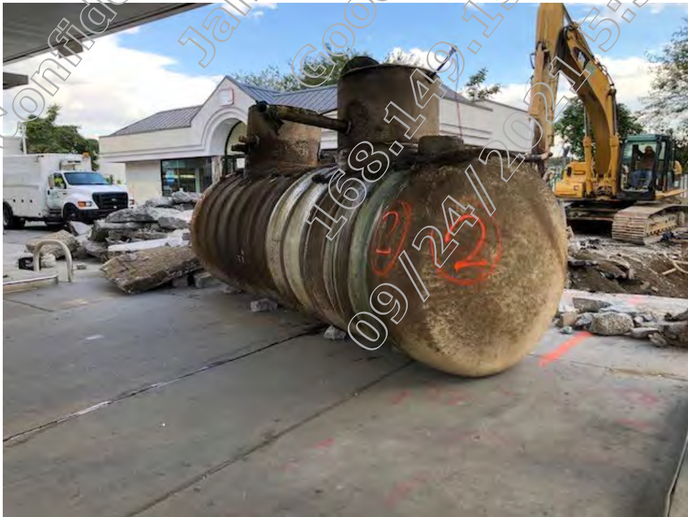
Condition of tank #2 (4,000-gallon double walled fiberglass)
