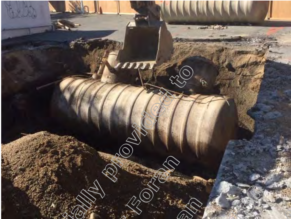
Removal of tank #4
