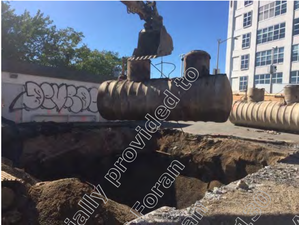
Removal of tank #5
