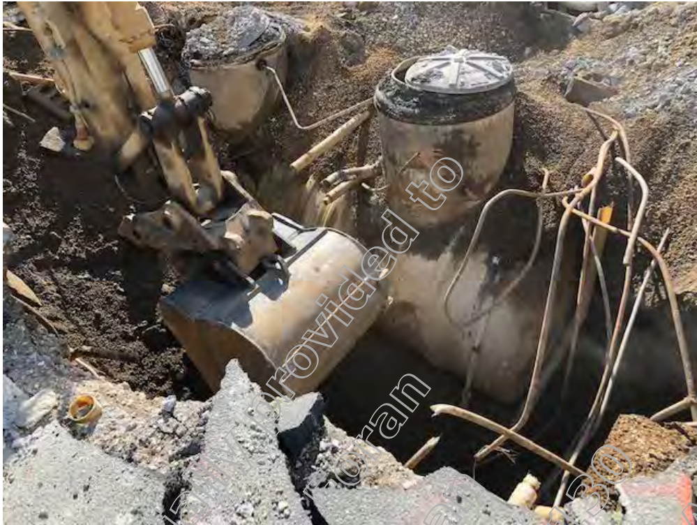
Excavating tank #1
