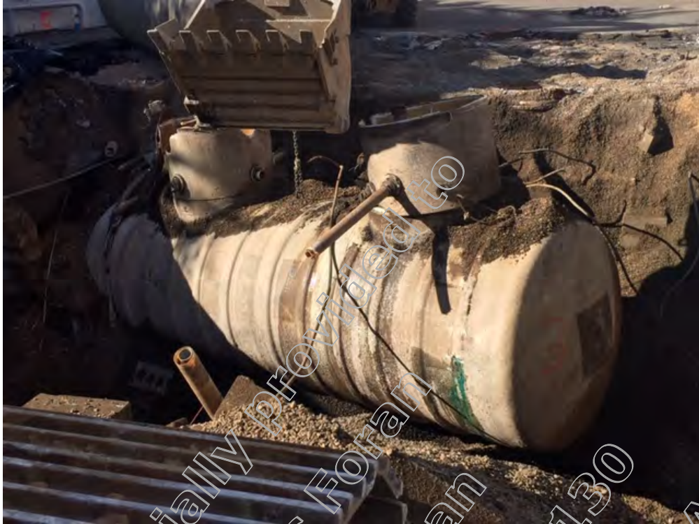
Removal of tank #3
