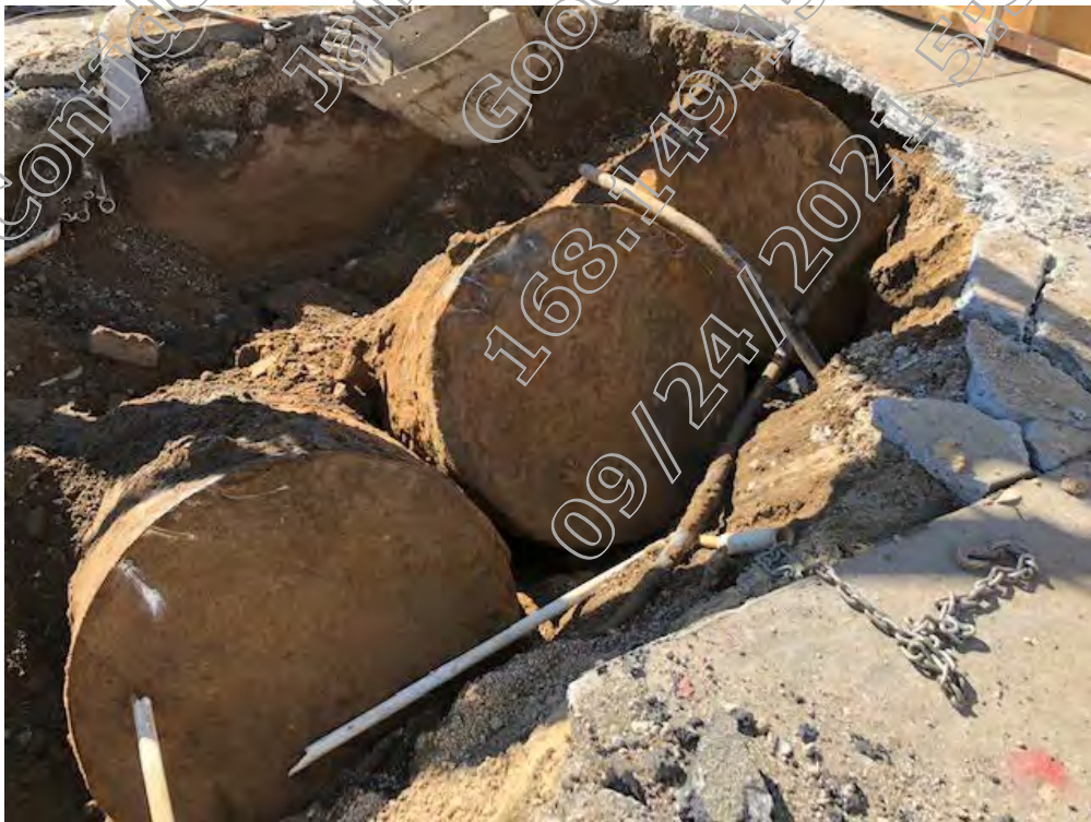
Remaining three 550 gallon capacity unknown tanks (no concrete encasement)
