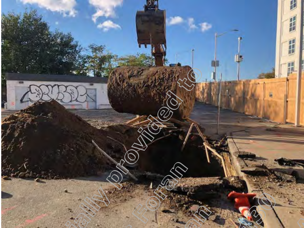
Removal of unknown tank #1 from excavation (550 gallon capacity)
