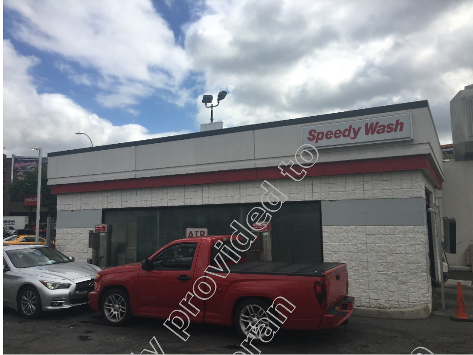
A view of the car wash located on the eastern portion of the subject property.
