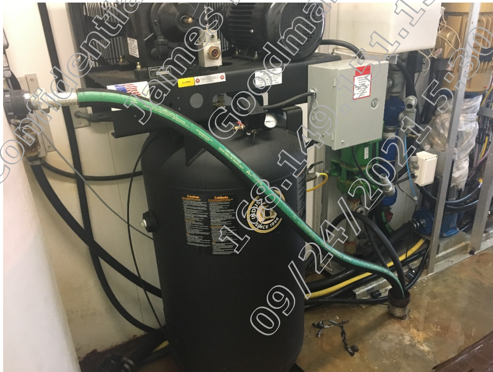
A 200-gallon tank for car wash detergent was located inside the car wash.
