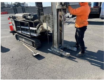
Photo 1: Lakewood advancing soil boring SB31 in the northern part of the site (facing southwest)
