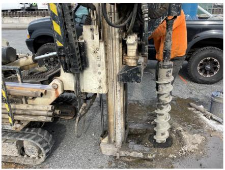
**Photo 2:** Lakewood using an auger to expand a borehole in preparation for monitoring well installation at soil boring SB21 (facing northwest)
