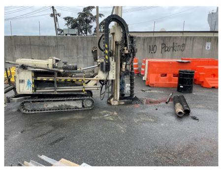
Photo 1: Lakewood using an auger to expand a borehole in preparation for monitoring well installation (facing east)
