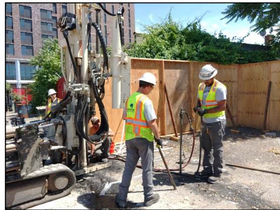
Photo 4: RRS field staff monitoring injections.
