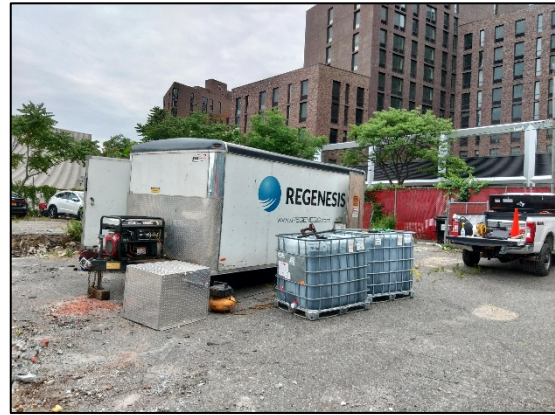
Photo 2: RRS Injection trailer onsite.
