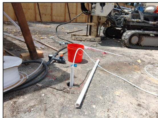
Photo 6: A temporary piezometer installed to gauge injection influence radius.
