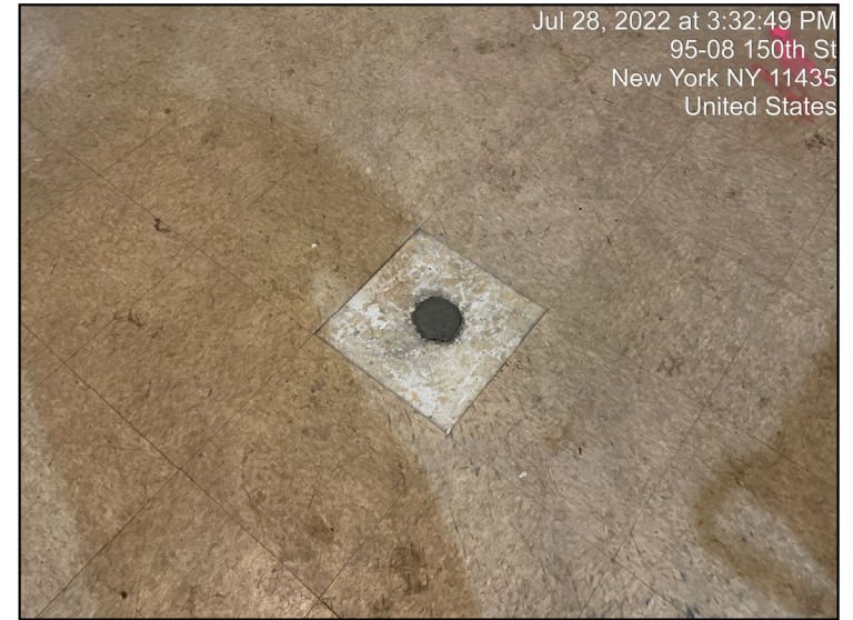
Photograph 10: Restoring Site conditions with cement patching.
