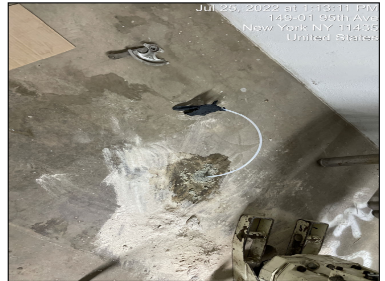
Photograph 4: Sub-slab soil vapor point installed at SV-06.
