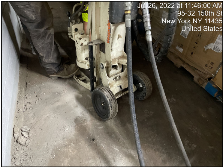
Photograph 5: Remote-access direct push probe at advancing RI-SB-09.
