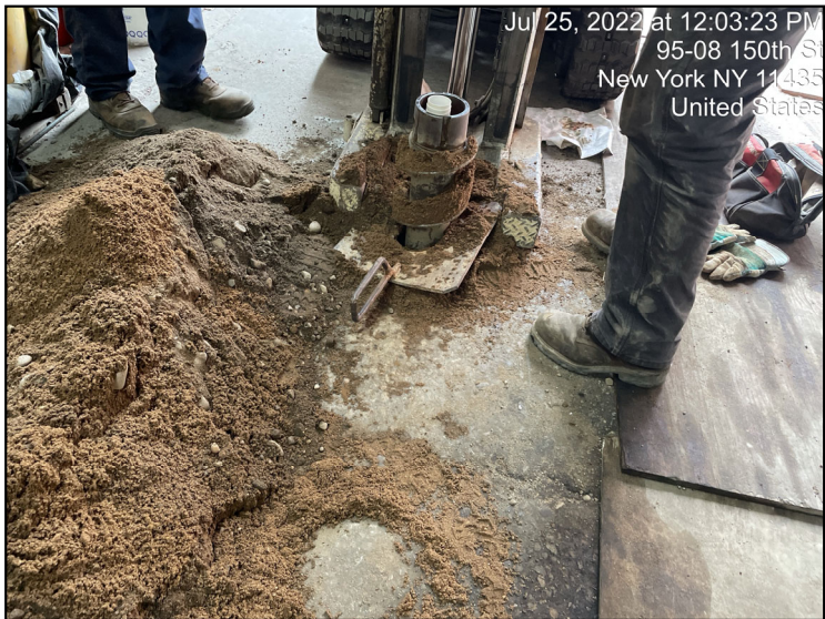
Photograph 3: Installing 2-inch PVC permanent monitoring well at location RI-MW-03.
