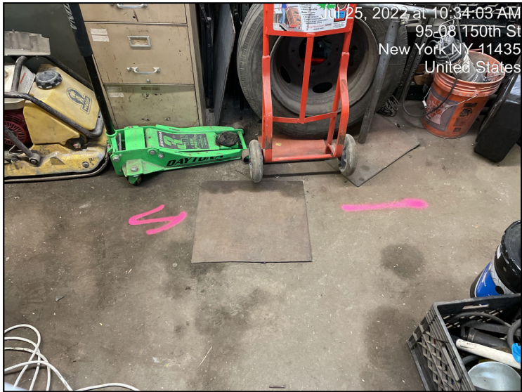
Photograph 1: Geophysical mark out near floor drain located on Lot 10 indicating potential subsurface piping.
