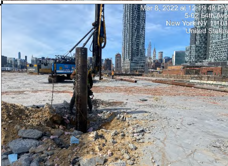
Photograph 2 - Index pile installation, facing west.
