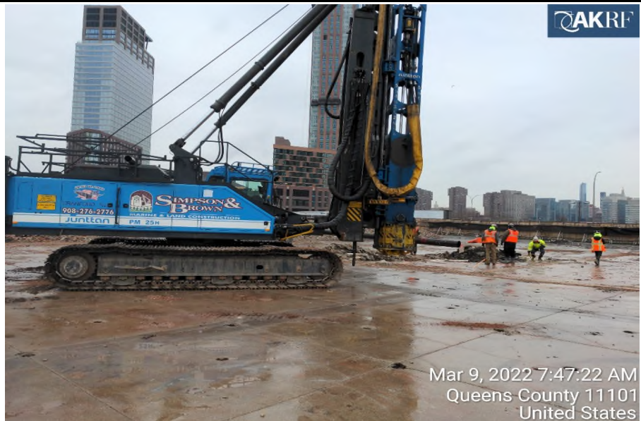
Photograph 3 - Index pile installation, facing south.
