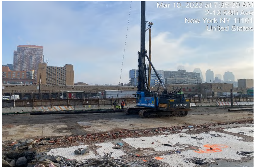
Photograph 2 - Index pile installation, facing north.
