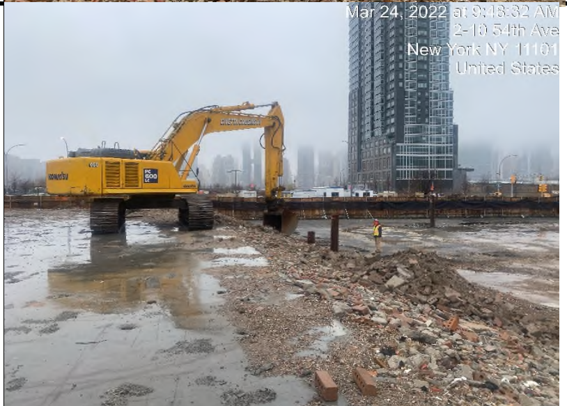
Photograph 2 - Civetta removing C&D from load testing location, facing west.
