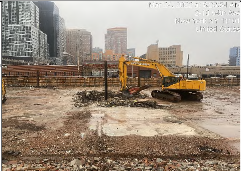
Photograph 1 - Civetta breaking up a portion of the former building slab in preparation for index pile load testing, facing north.
