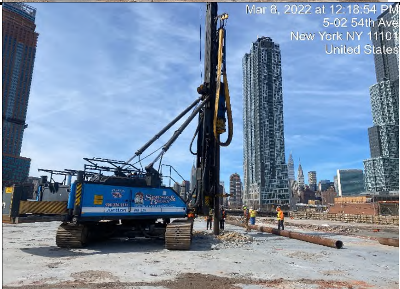
Photograph 2 - Index pile installation, facing west.
