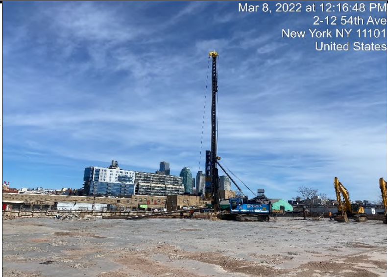
Photograph 1 - Index pile installation, facing northeast.
