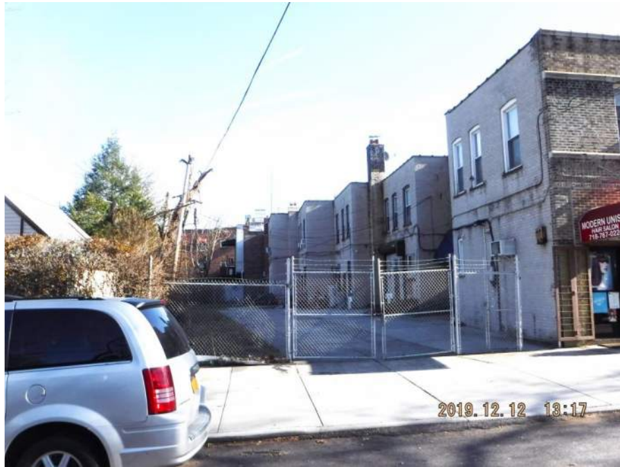
Photograph 1: General view of the rear Site yard looking east from 161 st Street. Site buildings at right.
