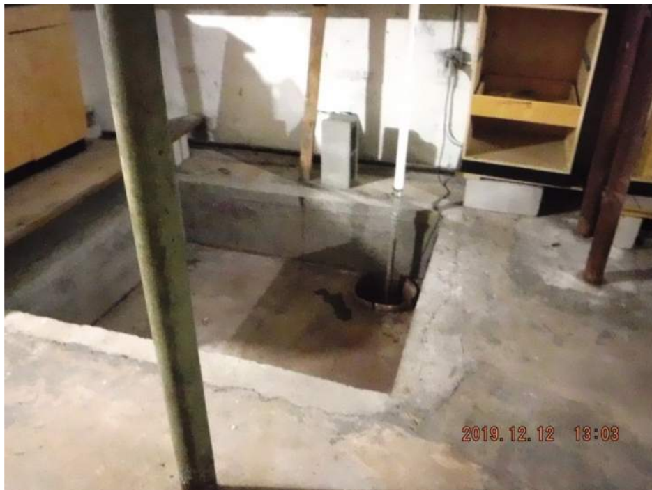
Photograph 4: Sump2 in the basement of 161-03 29 th Avenue.
