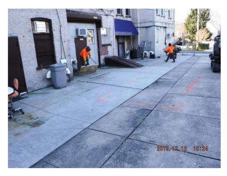
**Photograph 2:** Outline of the UST in red spray paint as established by the GPR survey. Photographer facing west.
