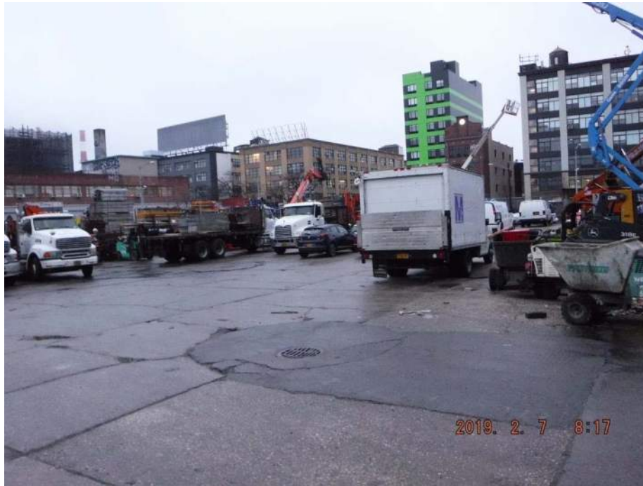
Photograph 3: General view of a portion of the Site stockyard looking north.
