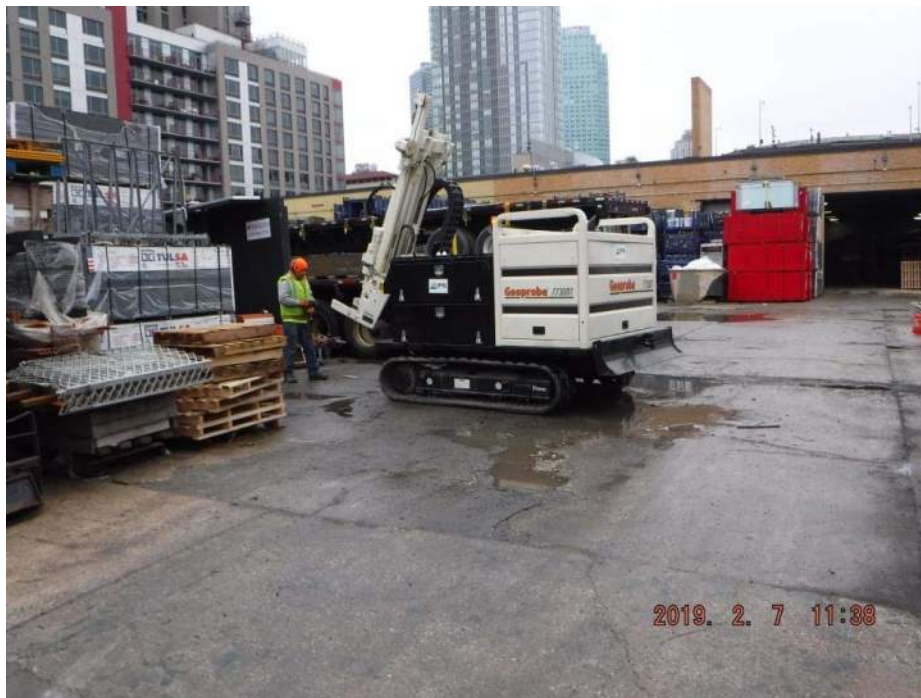
Photograph 4: Installation of B3 looking south.
