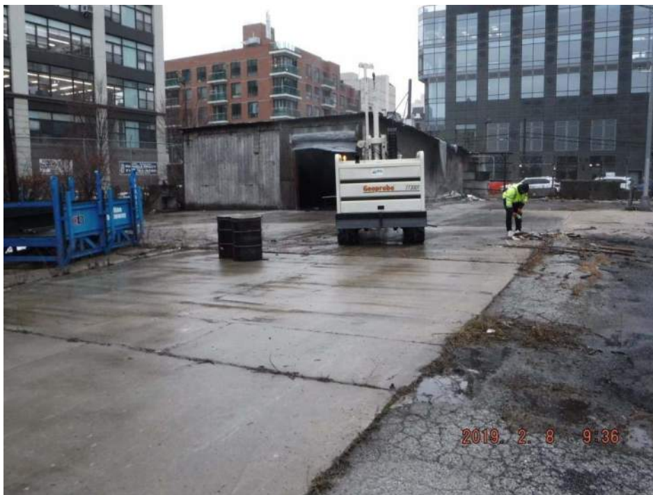
Photograph 8: Open and empty stockyard area at the north side of the Site looking east towards the vacant storage building.
