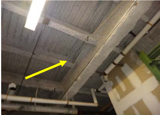
TYPICAL VIEW OF SUSPECT ASBESTOS SPRAY ON FIRE PROOFING ON SITE
