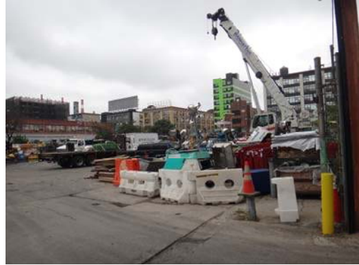
TYPICAL VIEW OF TENANT YARD AREA
