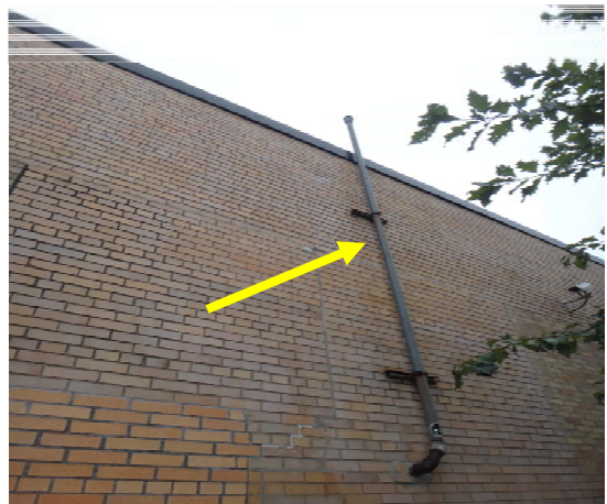
VIEW OF ABANDONED GASOLINE TANK VENT
