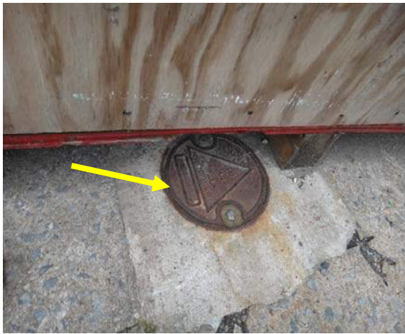
TYPICAL VIEW OF MONITORING WELL ON SITE
