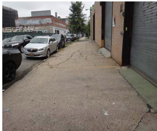
VIEW OF ROLL UP DOORS ON 23rd STREET
