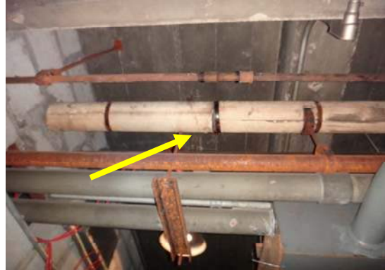
TYPICAL VIEW OF SUSPECT ASBESTOS PIPE INSULATION ON SITE
