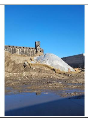
Photo 10: Stockpile covered with polyethylene sheeting and surrounded with hay bales, facing west. 03/21/2024.
