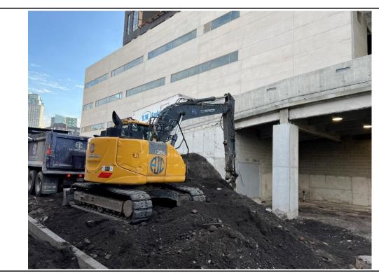
Photo 2: Excavator loading a truck with soil, facing northeast. Soil was not approved for off-site disposal. 03/20/2024
