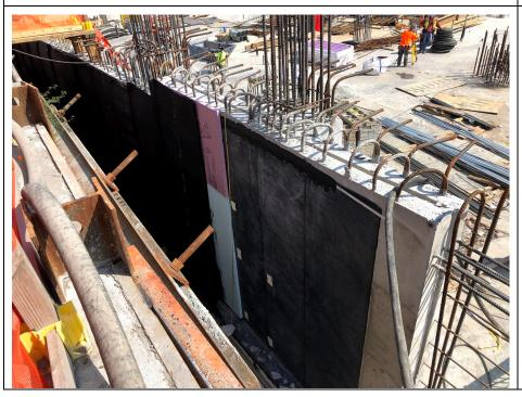
**Photo 4:** View of vapor barrier along the northwest foundation wall.
