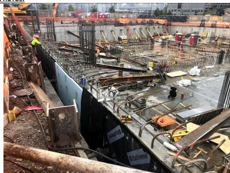
Photo 3: Looking north, view of New Leaf waterproofing the foundation wall along the southwest perimeter of the Site.
