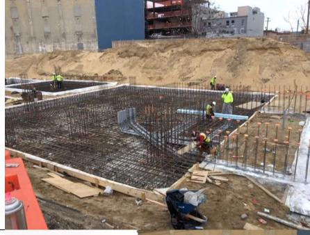
Photo 2- View of rebar installation in C6-C8.
