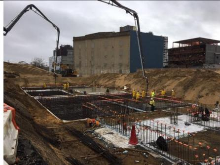
Photo 2- View of rebar and formwork installation in D1.
