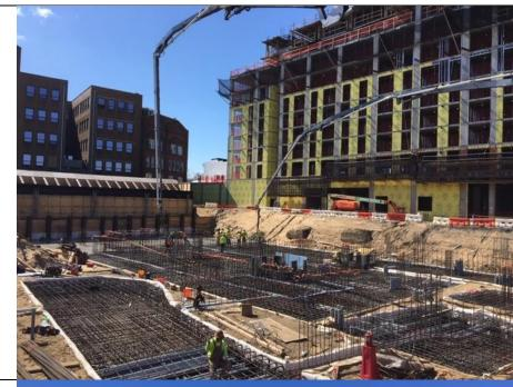
Photo 2- View of rebar, formwork, utility installation in A3, A4, B3, and B4.
