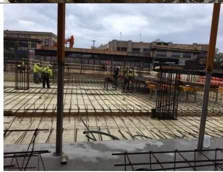
Photo 3- View of formwork, utility, and rebar installation in D3, D4, E3, and E4.
