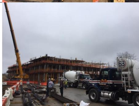
Photo 3- View of utility installation and pouring concrete in D3, D4, E3, and E4.
