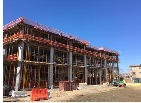
Photo 3- View of rebar, formwork, and utility installation in D3, D4, E3, and E4.
