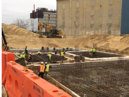
Photo 3- View of formwork and rebar installation in D1.
