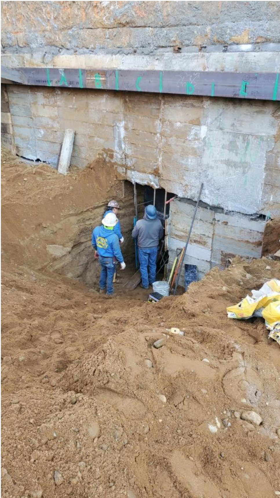
View of underpinning
