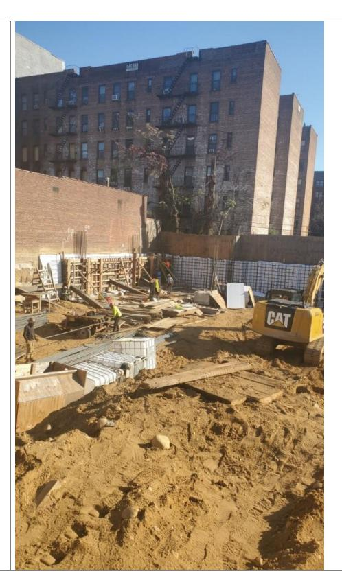
Photo 2-View of the Site where vapor barrier is being installed.
