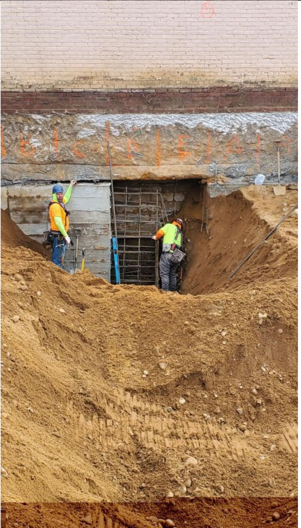
View of underpinning.
