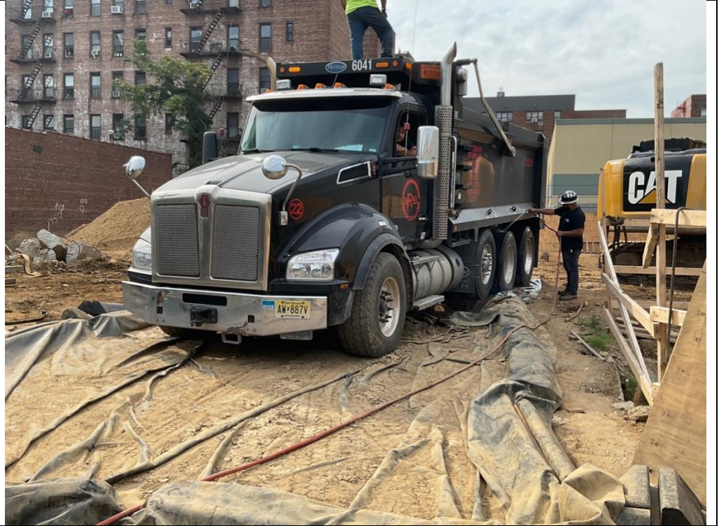
Photo 2 – Soil loading at the Site.
