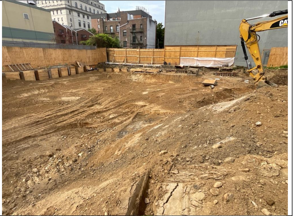
Photo 1 – An overview of the site towards the end of workday.
