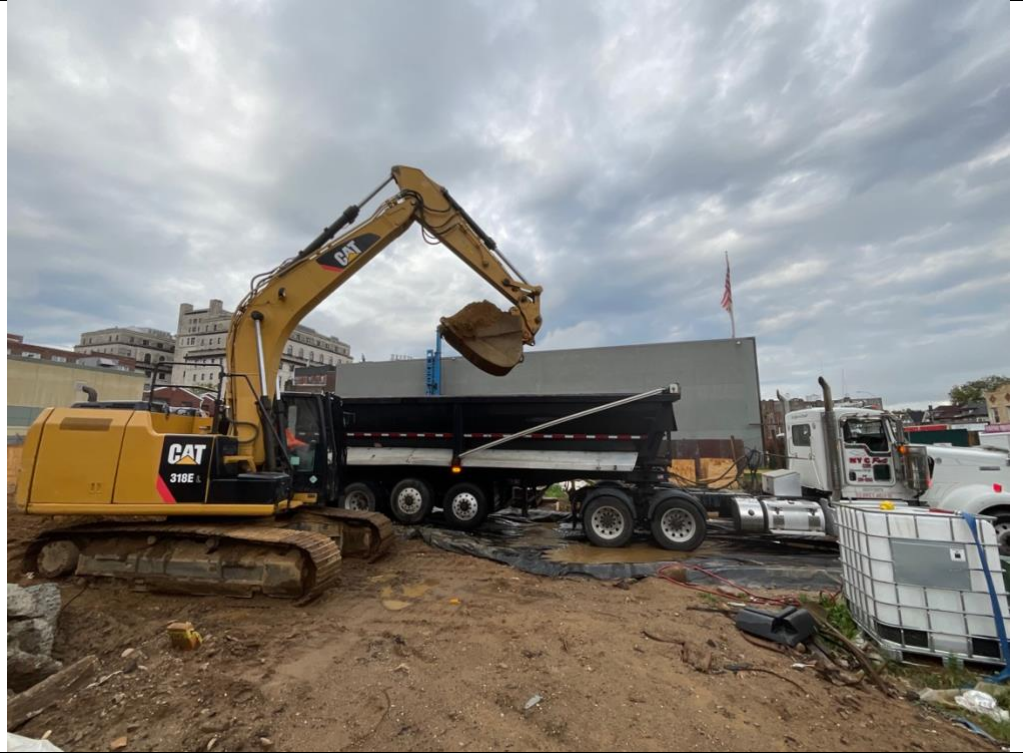
Photo 2 – Soil loading at the Site.
