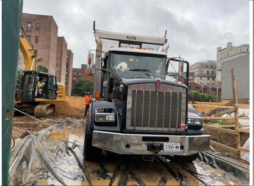
Photo 2 – Soil loading at the Site.
