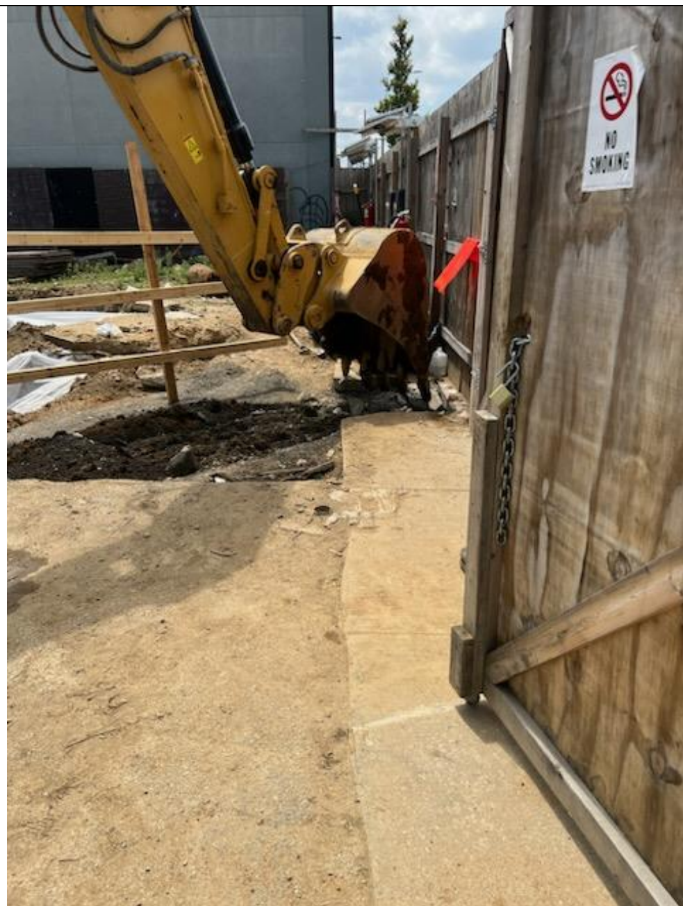
Photo 2 – Installation of test pit
