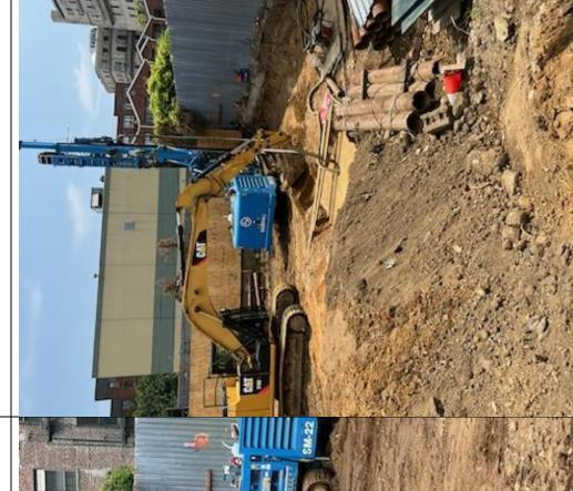
Photo 2 – Installing shoring piles along the southewestern perimeter of the site.
