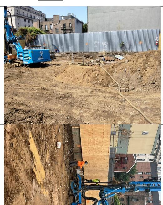
Photo 2 – Installing shoring piles along the southeastern perimeter of the site.
