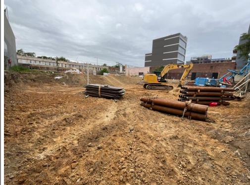
Photo 2 – Installing shoring pile in the SE corner of the site.
