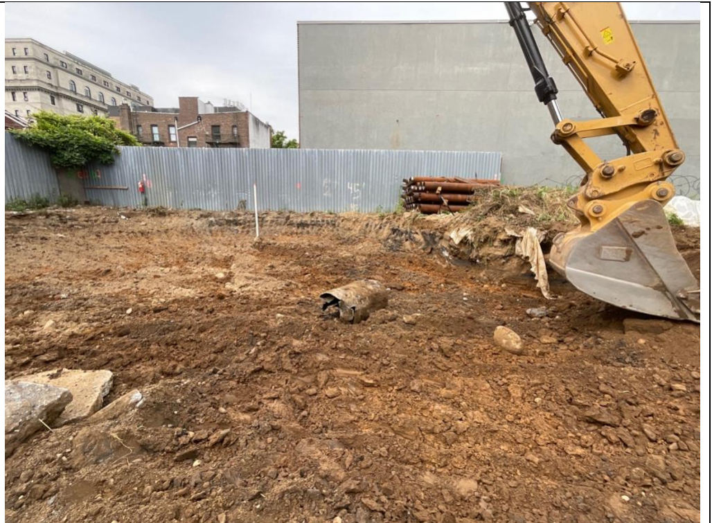
Photo 5 - An empty tank was discovered during the excavation in A3 & A4.
