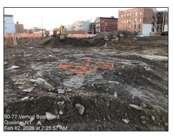
Photograph 6 – The hazardous lead-contaminated soil area was marked prior to excavation and removal (Feb 2020).
