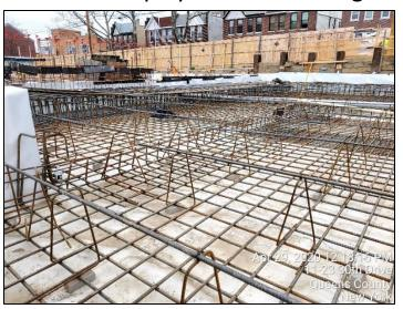
Photograph 10 – Installed GCP Preprufe 200 vapor barrier/waterproofing membrane below the foundation slab and behind subgrade foundation walls (April 2020).
