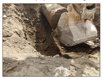
Photograph 2 – The tank was removed following removal of the oil-water mixture (October 2018).
