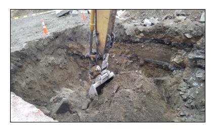
Photograph 4 – Petroleum-contaminated soil was excavated and removed following the tank removal (October 2018).
