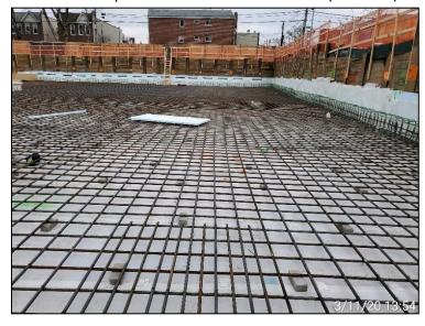
Photograph 8 – Installed GCP Preprufe 200 vapor barrier/waterproofing membrane below the foundation slab and behind subgrade foundation walls (March 2020).
