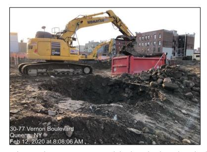
Photograph 7 – Excavating and loading the hazardous lead-contaminated soil (February 2020).
