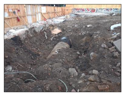
Photograph 1 – The underground storage tank (UST-1) was exposed for cleanup and removal (October 2018).
