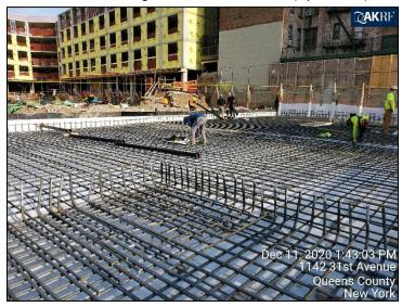
Photograph 12 – Installing the vapor barrier below the slab (December 2020)
