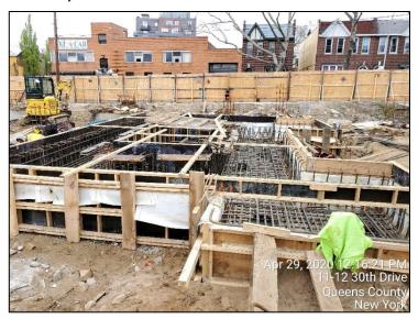
Photograph 9 — Installed GCP Preprufe 200 vapor barrier/waterproofing membrane below the foundation slab and behind subgrade foundation walls (April 2020).
