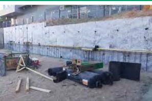
**PRECON** is comprised of a non-woven fabric, elastomeric membrane and **W. R. MEADOWS'** exclusive, patented plasmatic core (U.S. Patent No. 7,179,761). The plasmatic core is a seven-layer matrix designed for toughness and provides the lowest water vapor transmission (WVT) rating on the market. Designed to provide a waterproof seal between the membrane and poured concrete, **PRECON** also:
