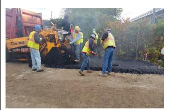
Photograph 9 2" Asphalt Cap at Cap Area 1.
